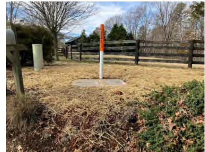
Completed underground vault installation in central Virginia, Albemarle County. Fiber drops to the home will connect to this point.
