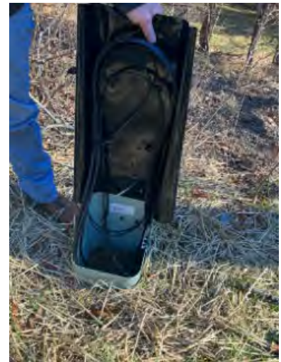
A broadband network terminal, where lines are connected between line extensions to households and mainline broadband infrastructure
