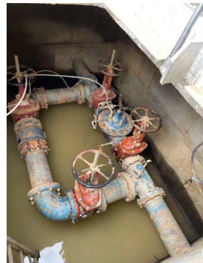
Flow control valve vault which allows water to flow into town from near the spring and the upper side water storage tank.
