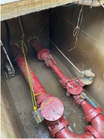
Altitude valve vault at one of the town water storage tanks. This tank would not fill completely.
